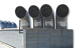
With normal use, commercial kitchen exhaust systems accumulate a flammable combination of atomised oil, fat and grease. Without regular duct cleaning, this residue can increase to become a significant fire hazard.
